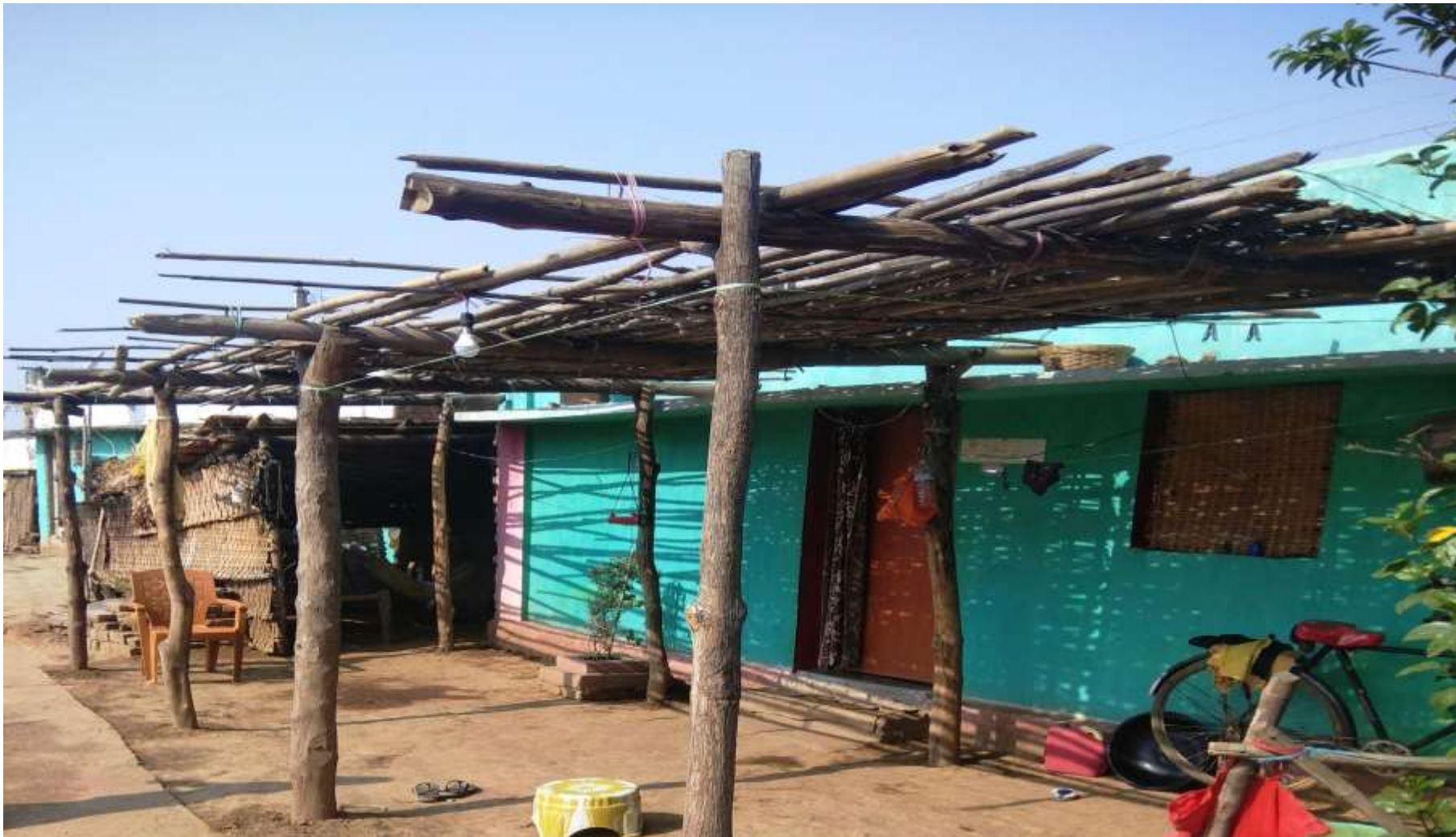
Figure 21: In the social supply chain, the forest fringe communities access forest bamboo as nistar to meet their bona fide needs such as fencing, roofing, shade, housing, utility items etc. Aspiration for pucca houses and promotion of brick masonry houses in government housing schemes has reduced the demand for bamboo in the housing sector
